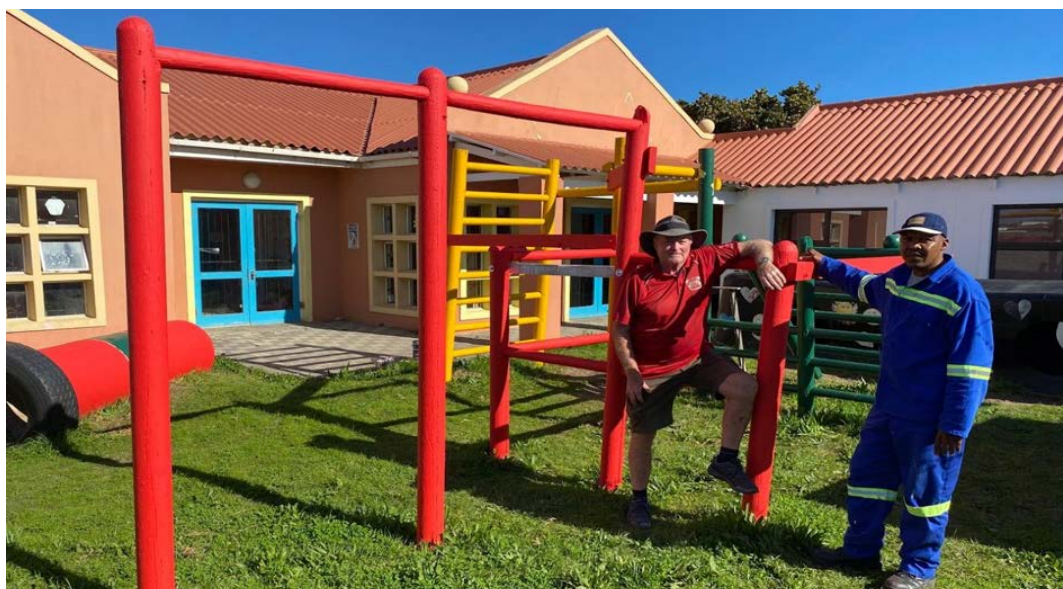
OGG member John Atkinson and Tshepo (our local painter) repairing playground apparatus at Nomzamo ECD School in Zwelihle Township, Hermanus (June 2026)
